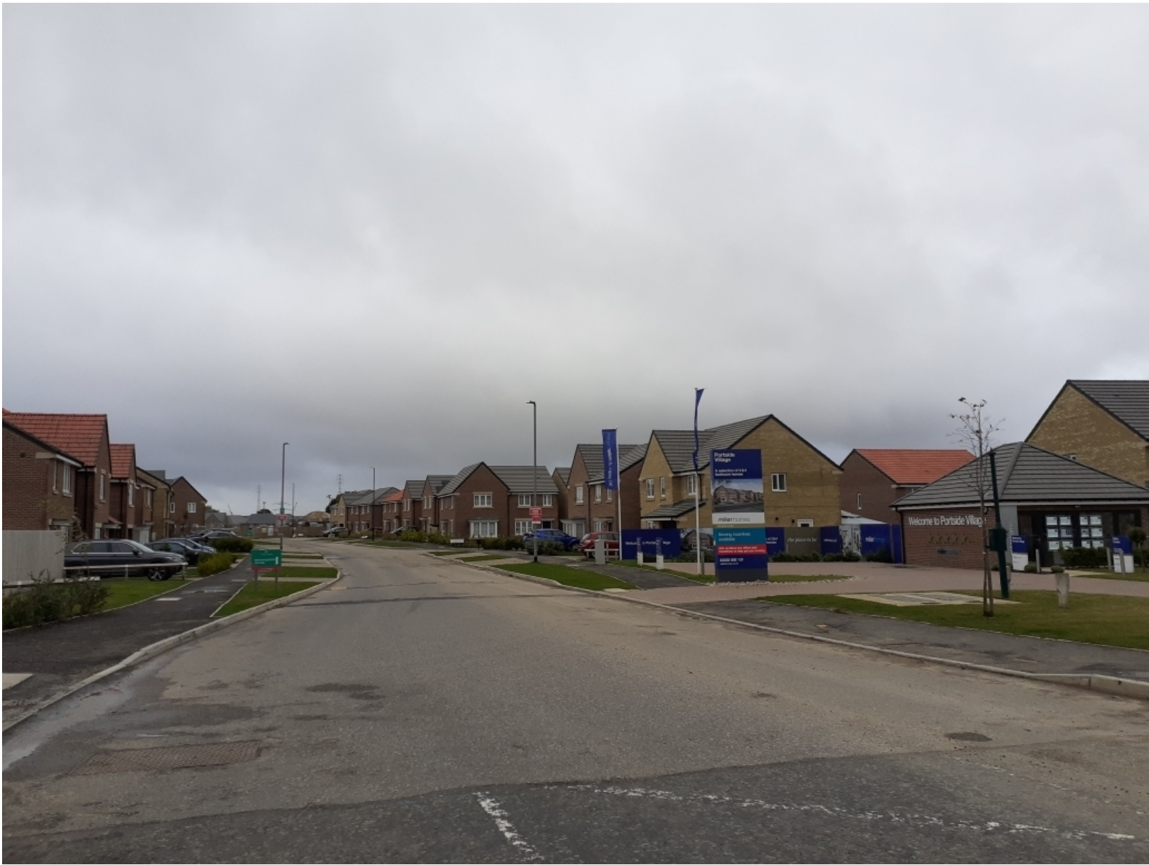
R/2024/0196/RMM Land at Low Grange Farm, South Bank Photographs
